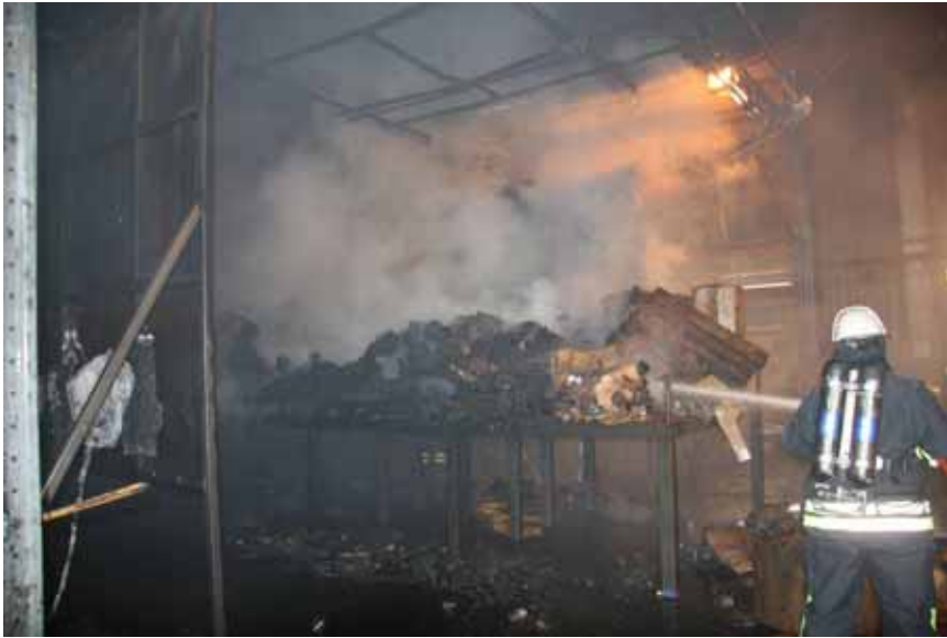
Figure A-80 Test 7E(HP-5.8): The fire damages, as seen from the left hand side, after the removal of the fire damaged pallet loads of commodity at the back end.
