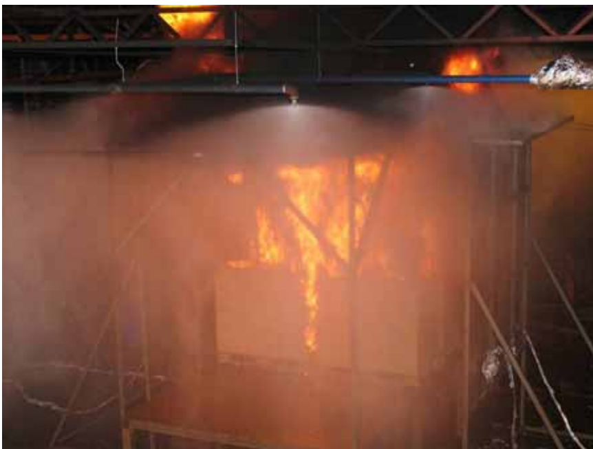
Figure A-123 Test 3S(10): Photo taken at 02:29 [min:sec] after fire ignition, at the moment the water spray system was manually activated.
