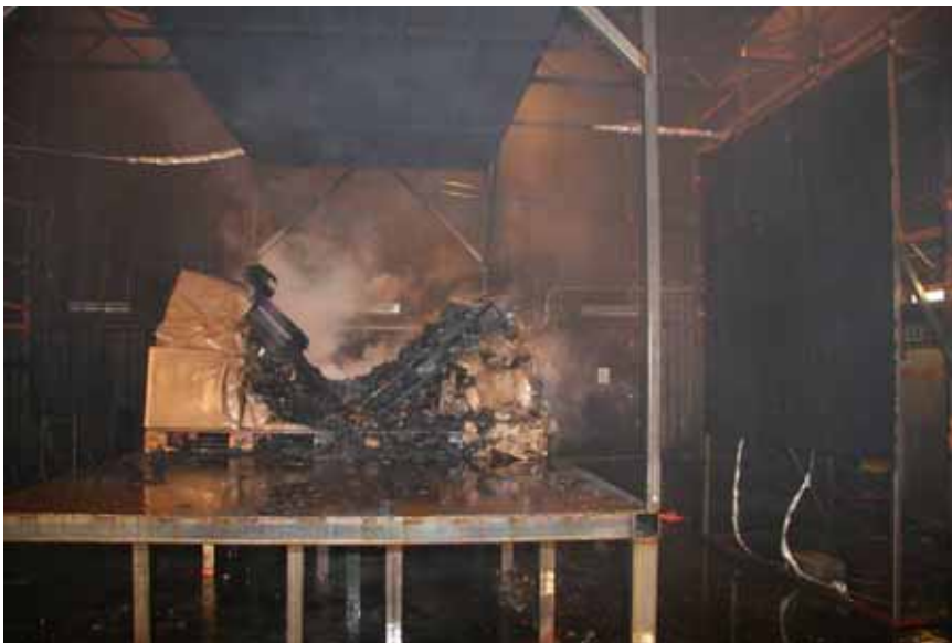
Figure A-127 Test 3S(10): Fire damages as seen from the back.
