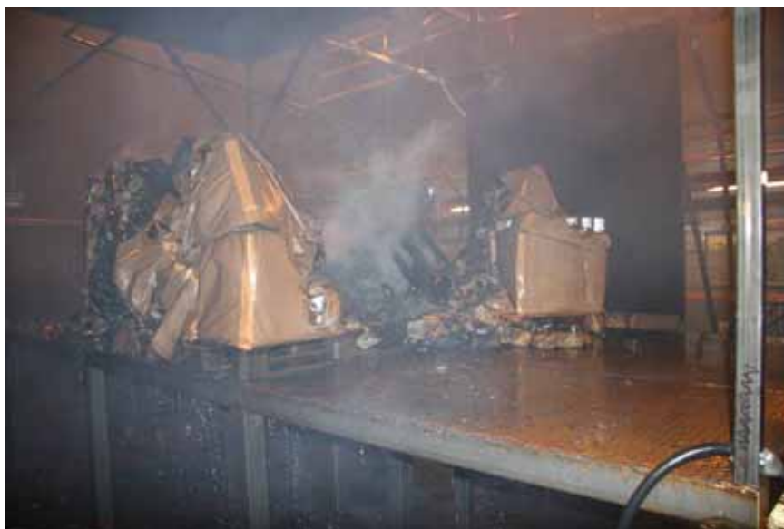
Figure A-116 Test 2S(10): The fire damages, as seen from the left hand side.
