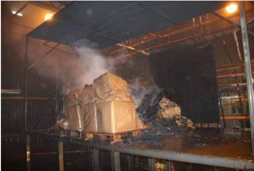
Figure A-128 Test 3S(10): Fire damages as seen from the left hand side.
