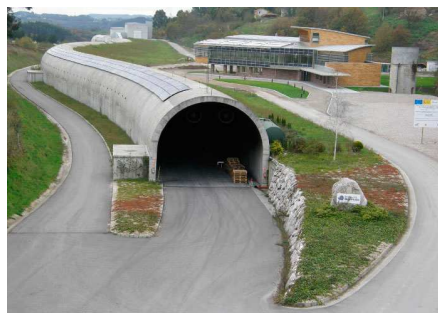
South portal of the tunnel
