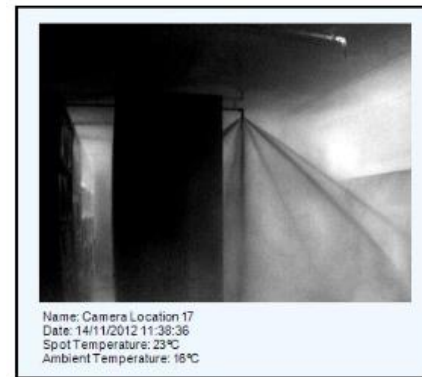
Thermal image of aisle nozzle discharge post fire brigade intervention. Location right of rack A as taken from pump set using one of the hand-held thermal imaging cameras.
