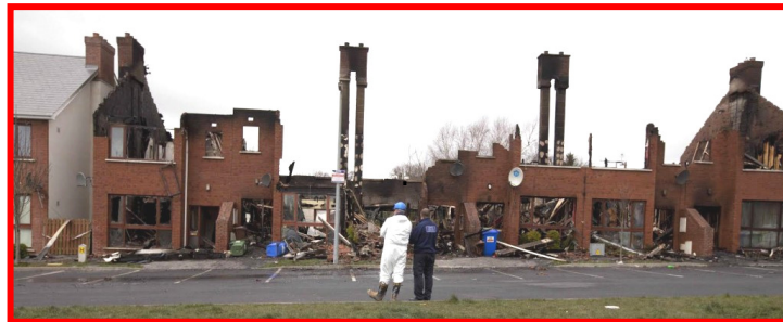
Timber-Framed Housing, Ireland 2015-03-31
