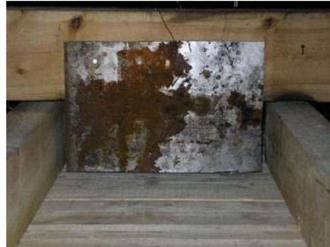
Detail of the plates installed to partially close the channel gaps
