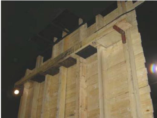
Detail of the plates installed to partially close the channel gaps
