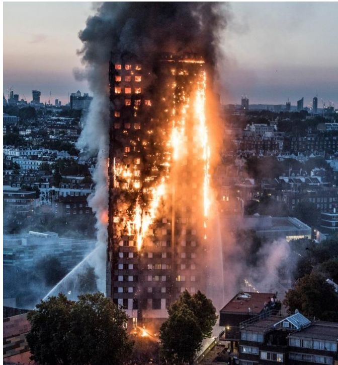
Grenfell Tower, London, UK, 2017 The Telegraph
