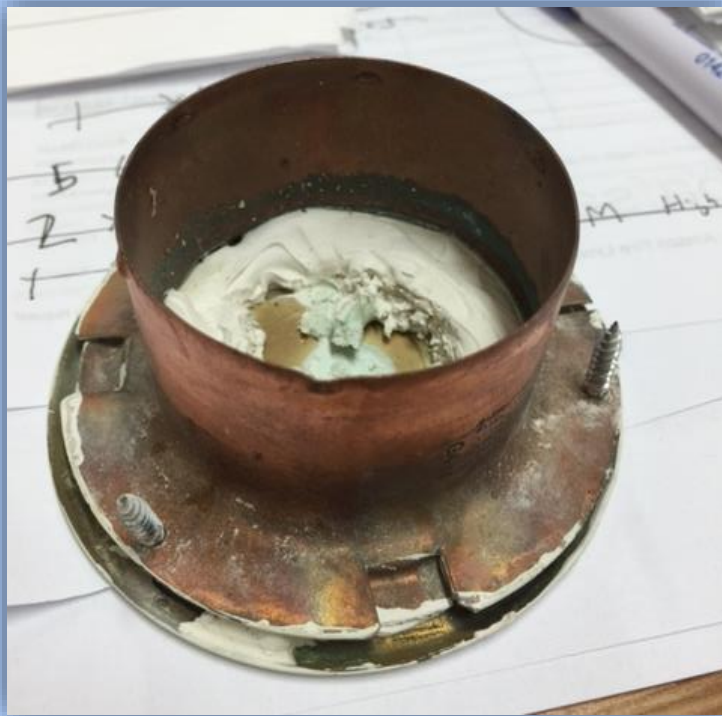
Plaster closing air gap
