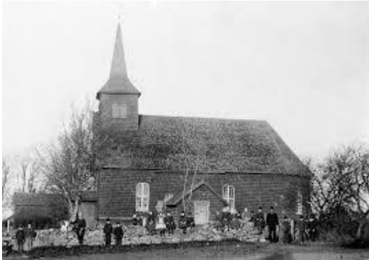
Älgårds church, Sweden. A rare, medieval wooden church (C15), protected internally and externally with an Ultra Fog water mist system.
