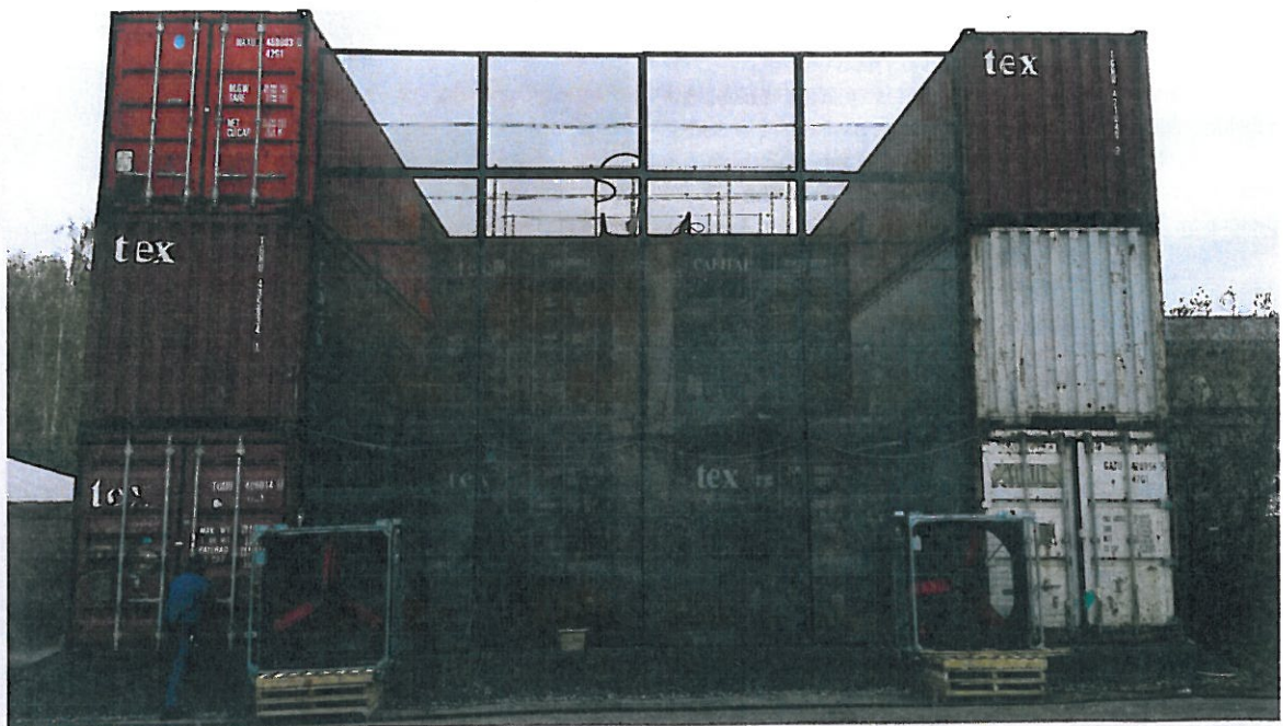
Fire-test rig built by Fogtec to prove the effectiveness of water mist for Dubai's new large-scale substations.
