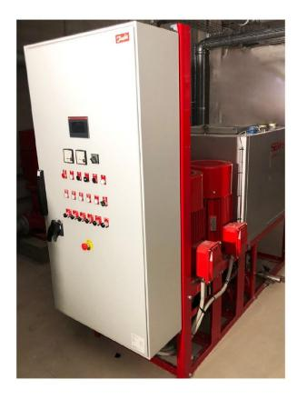
"The technology chosen to protect specific areas in the Regional Hospital Gødstrup is the SEM-SAFE® high-pressure water mist firefighting system. It comprises a high-pressure modular pump unit, section valves, piping and water mist nozzles. Apart from that we have supplied two SEM-SAFE® high-pressure water mist pump units, each with four pumps, 120 kilowatt working in a master-slave configuration and an integrated flow test system controlling 52 sections", says Henrik Bygbjerg.
