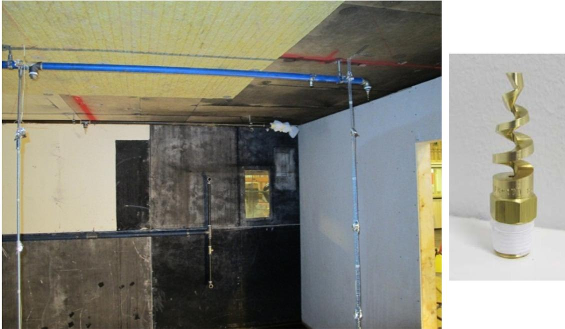
*Figure 5 Low pressure water mist system. Parts of two of the longitudinal pipes and four nozzles are shown. Close-up of the BETE TF8-170 nozzle is shown on the right.*
