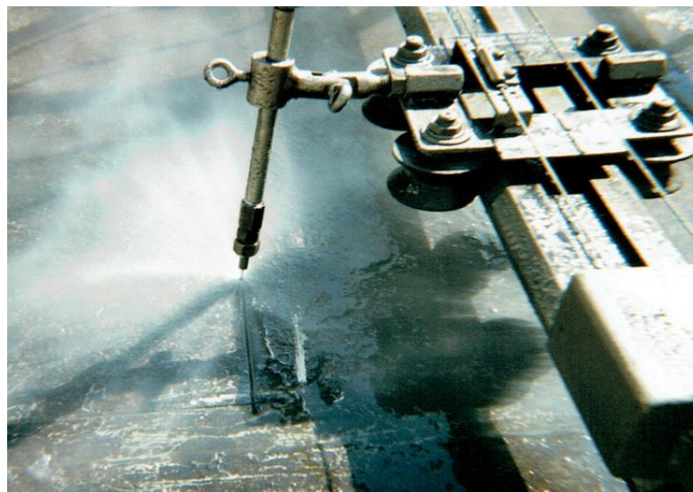
Opening man-hole in oil tank
