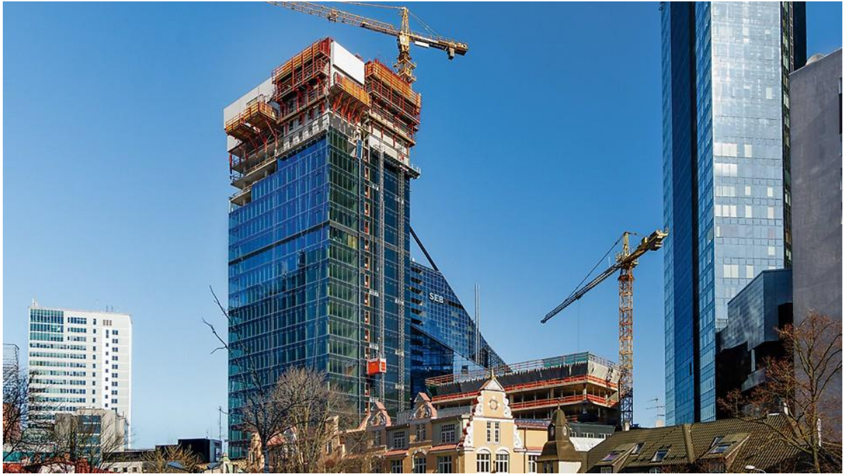
Maakri Tower (still under construction)
