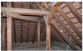
A fire risk assessment determined the need for an active fire fighting system in the attic space due to the exposed wooden roof support structure, no fire compartmentation and air conditioning equipment being located in the attic space
