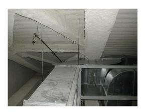
Risk of severe damages to of the gypsum theatre ceiling with precious paintings and frescos or even its collapse if conventional sprinklers would have been used to protect the attic space (soaking of water into the gypsum ceiling)
