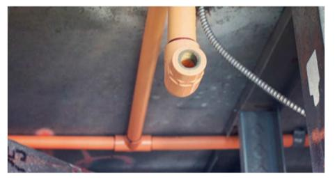
...certainly performs very well against corrosion but is not suitable for dry or higher pressure systems
