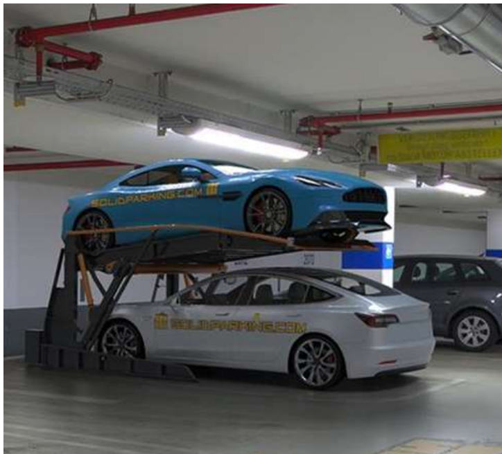
Fig. 2 Example of a two-tier car stacker. Source: solidparking.com
