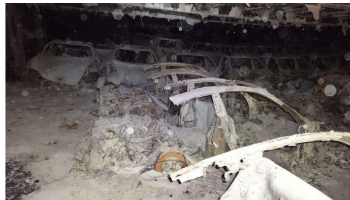
Fig. 20 Fremantle Highway – cargo hall post fire view
