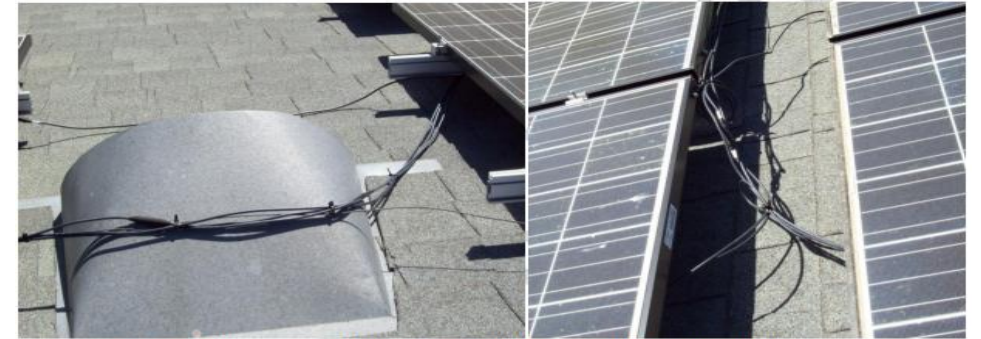
Figure 9 improper cable support with exposure to physical damage
