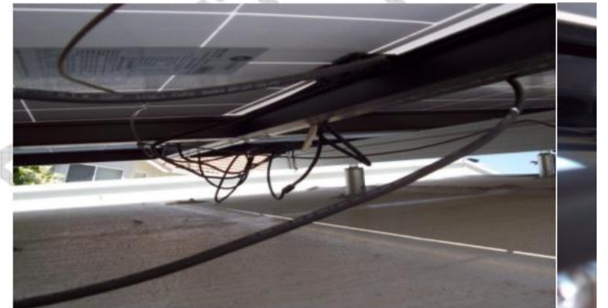
Figure 10 poor conductor handling and bending radius too tight
