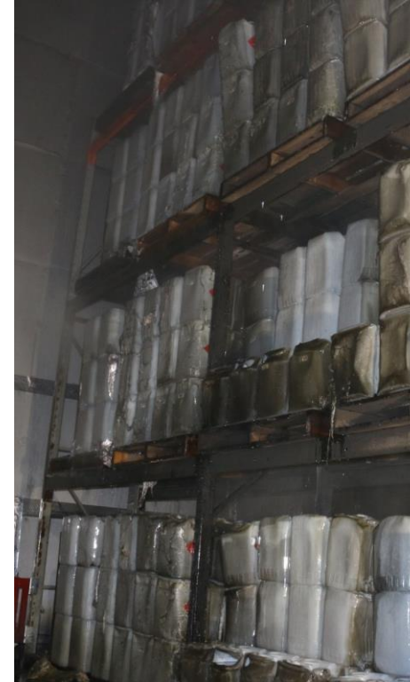
Main fuel array, 4-tiers 49 containers breached
