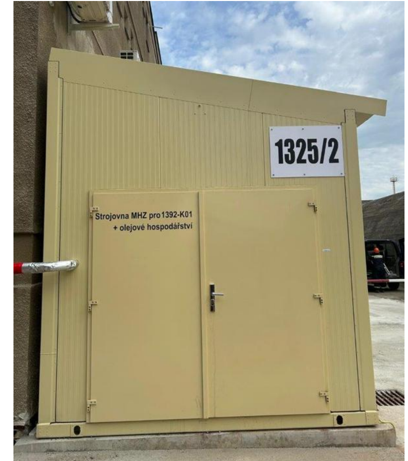
External view of the technological house
