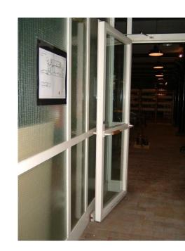
Solution: water mist in combination with 30 min resistance to fire
