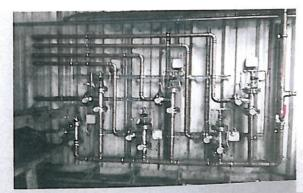
The system consists of six control valves and two full-duty pumps (plus one for pressure maintenance).
