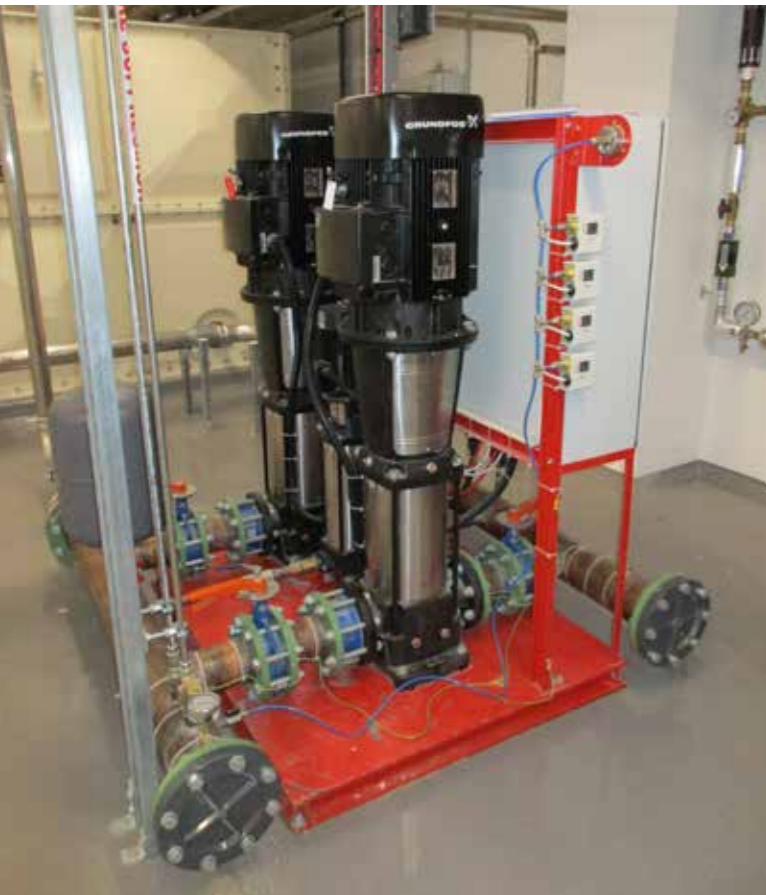
◀ Example of a small pump and water tank – a benefit for watermist. Image courtesy of VID Fire-Kill.
